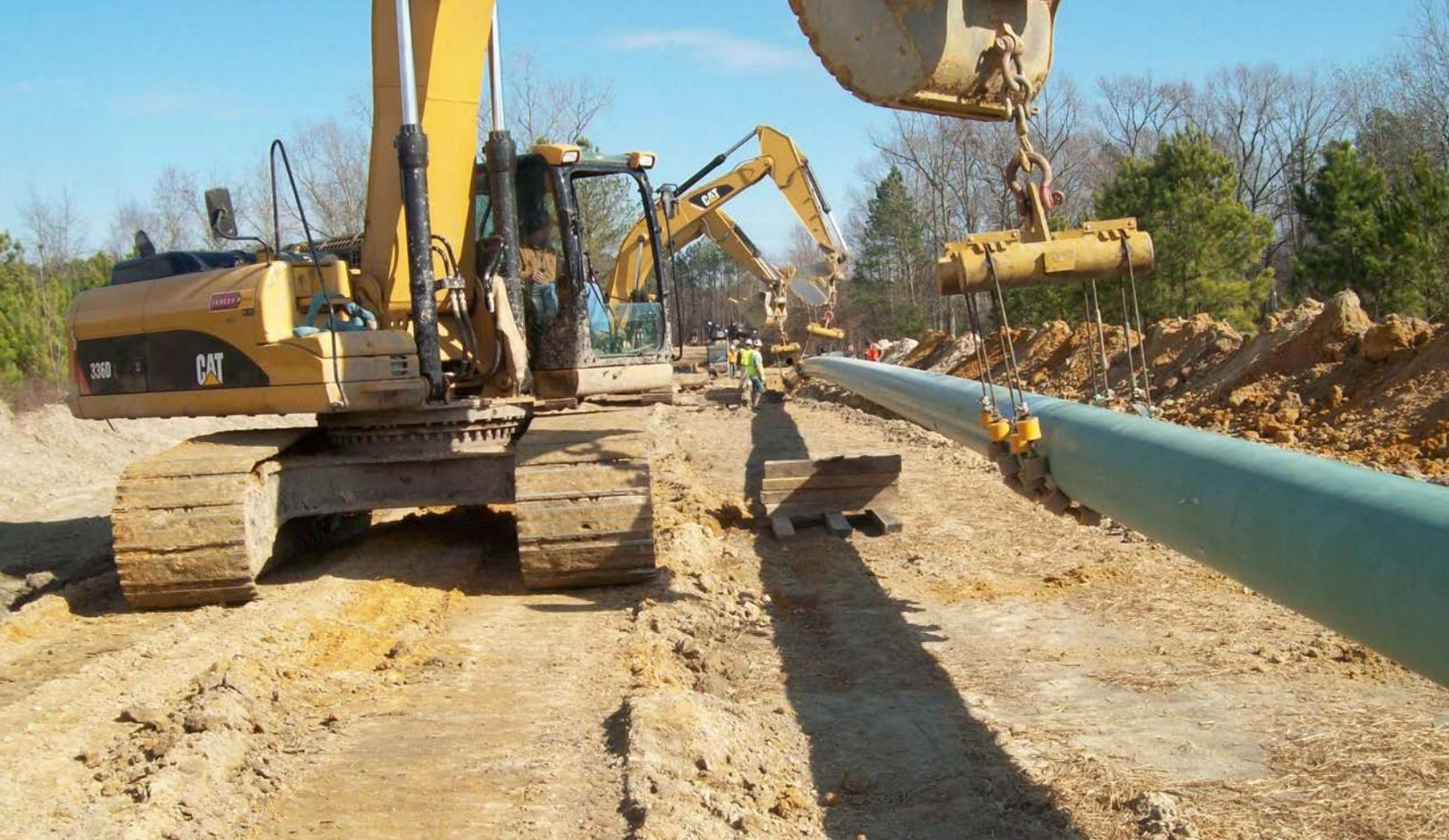
such as open ditches, ditch collapse hazards, crush injury hazards (pipe can weigh hundreds of pounds per foot), heavy equipment operations, overhead electrical hazards, etc. A project safety manager will be assigned but safety is the responsibility of every person on the line.
