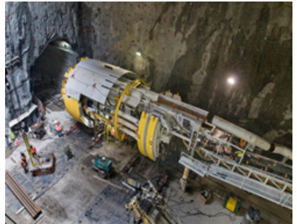
Tunnel Boring Machine
